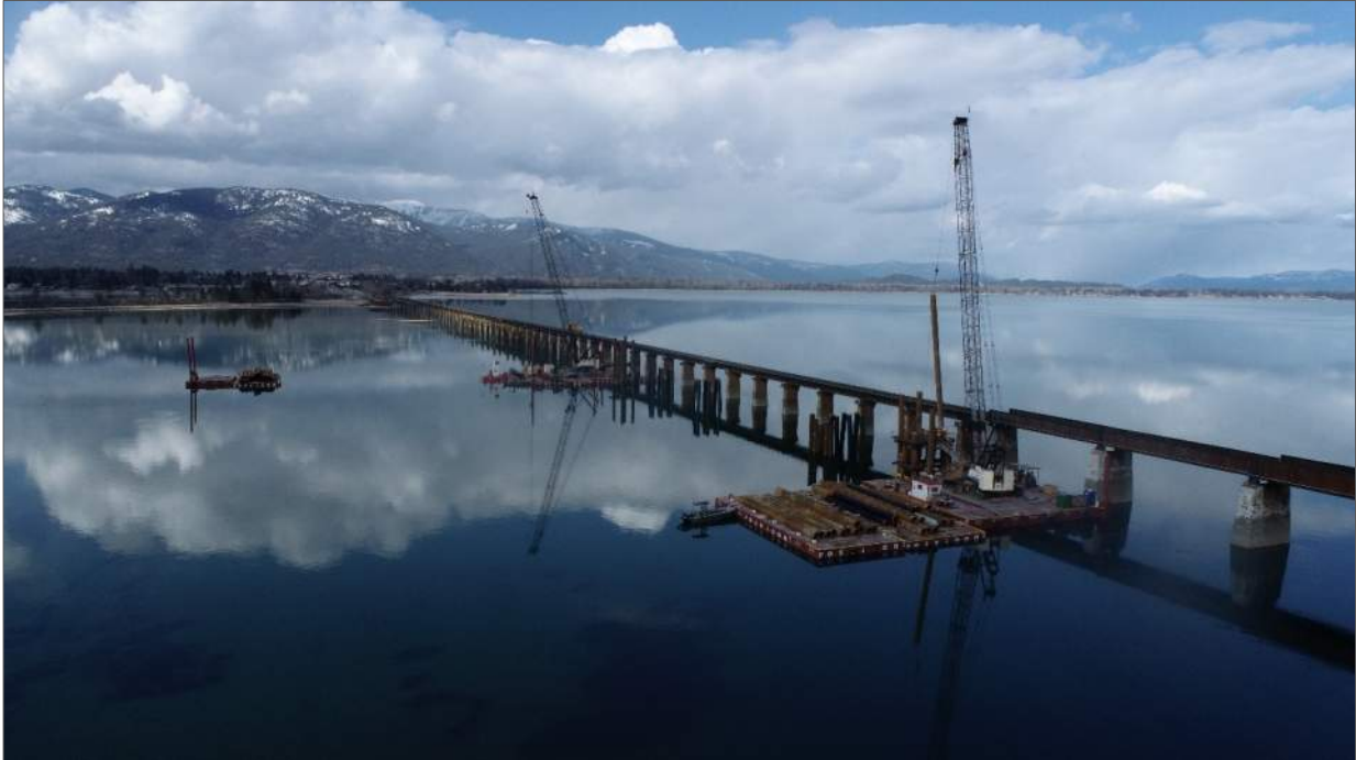
Photograph 3: Drone photograph including barges constructing new bridge.
