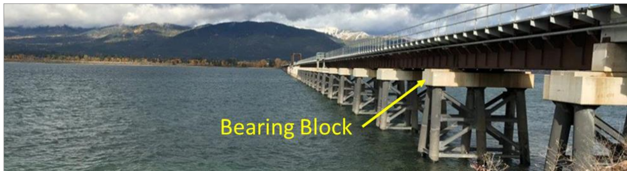
Photograph 1: Concrete Bearing Blocks on Existing Bridge 3.9E
