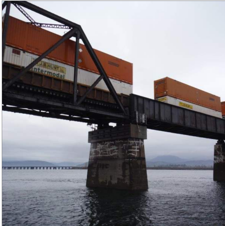
Figure 3: Bridge Pier Photograph
